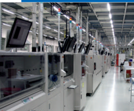
Complete Solar production line at Asys
